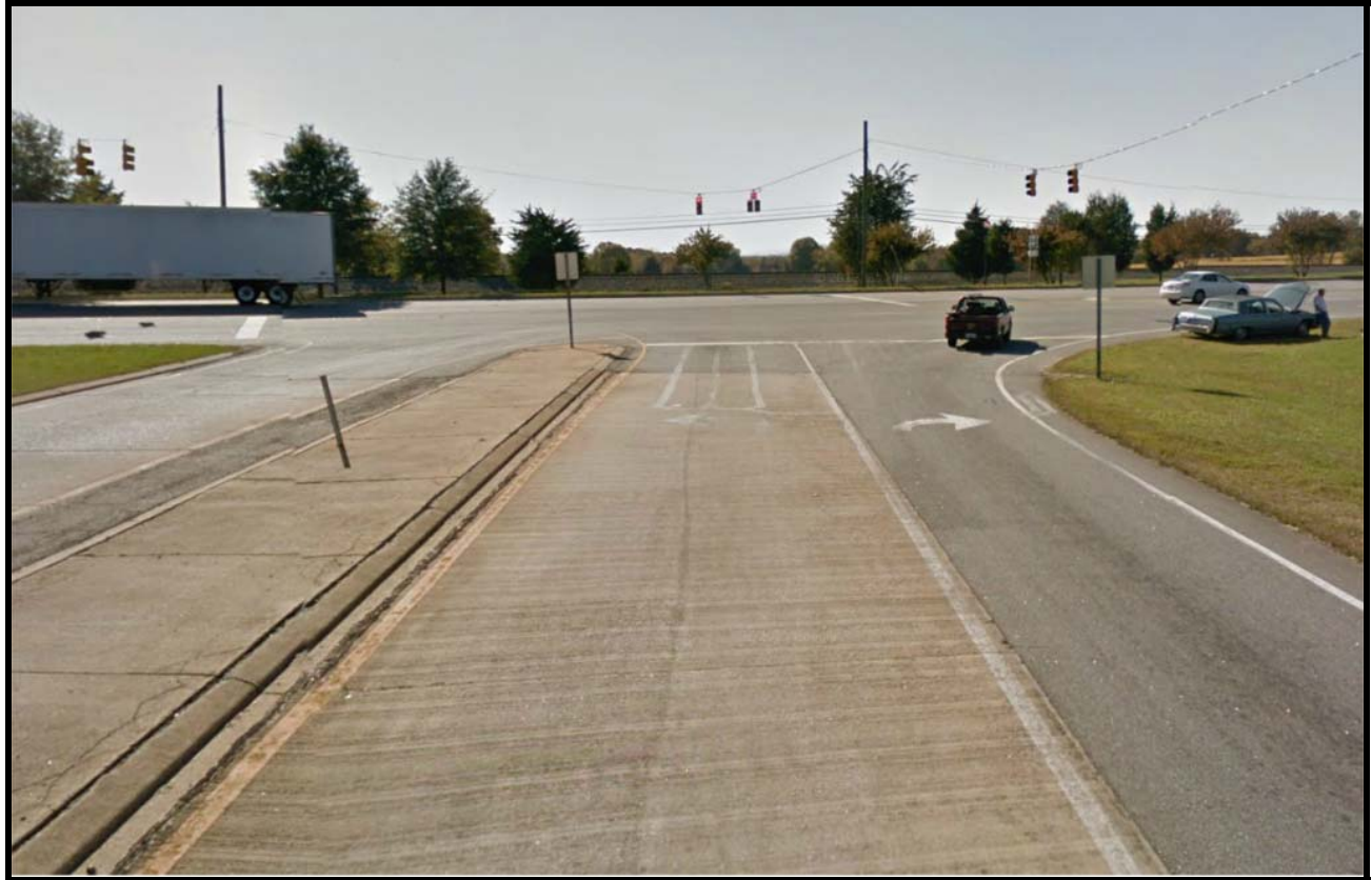
Google Maps (October 2012) – Looking West on I-40 Westbound Off-Ramp
